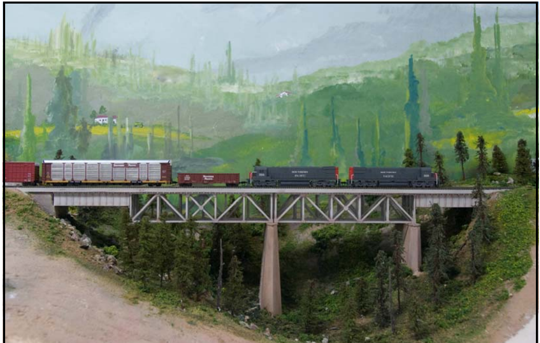
Butte Canyon Bridge near Cisco, California
